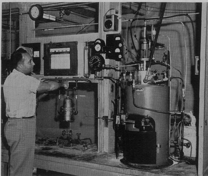
Figure 1. Reactor for production of ammonium polyphosphate from superphosphoric acid and ammonia
